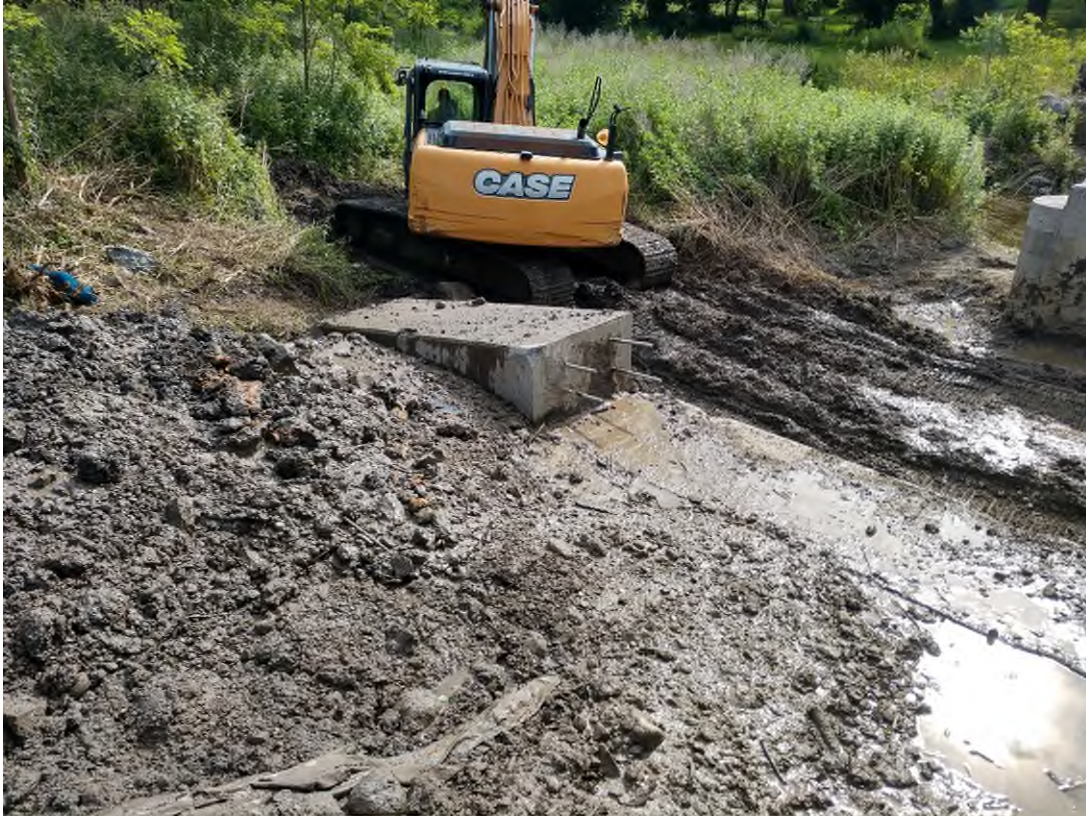
East Sherman Hollow – New abutment cap with dowels, West side
